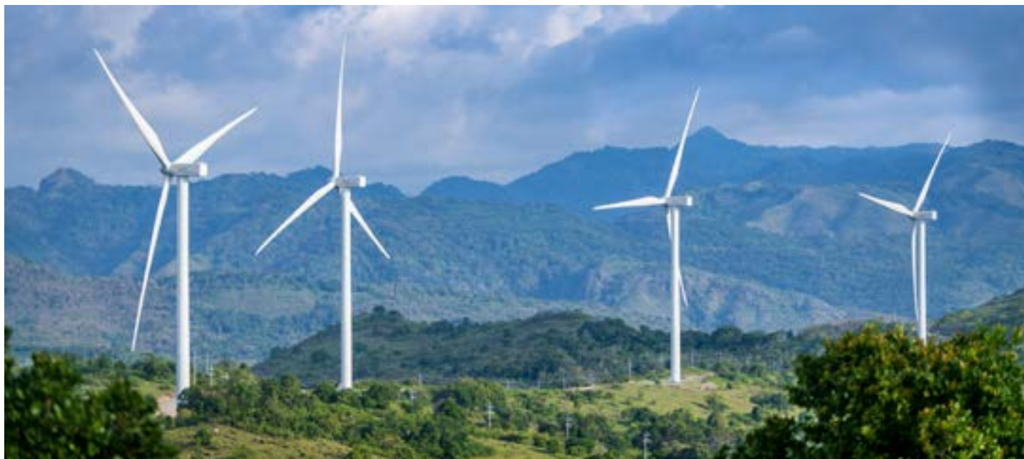
Indonesia's first commercial-scale wind farm was inaugurated in Sulawesi in 2018 with $120 million in financing from OPIC. (Credit: OPIC)
